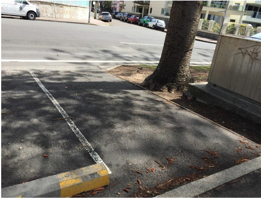
Figure 5: Opposite 72 North Steyne, Manly
