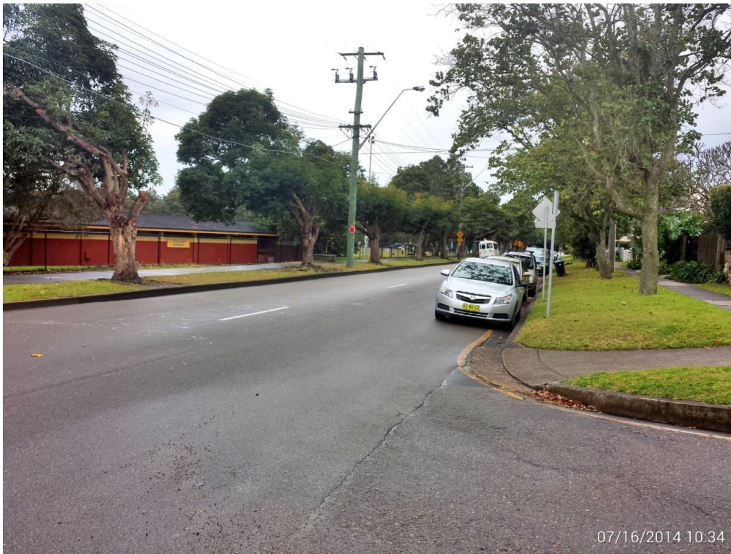
Figure 1: View East (Right Hand Side) of Balgowlah Rd from Daintrey St; restricted sight distance for westbound traffic.
